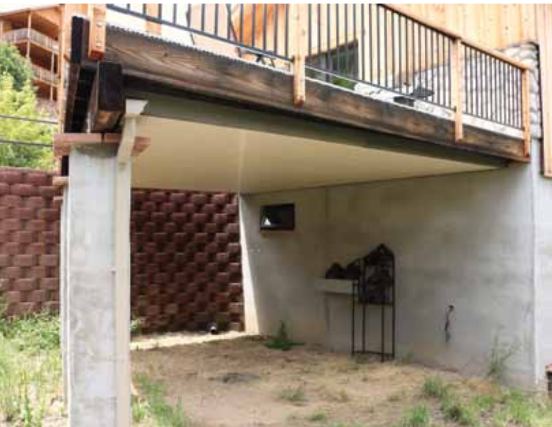
After Installing TUFTEX DeckDrain
